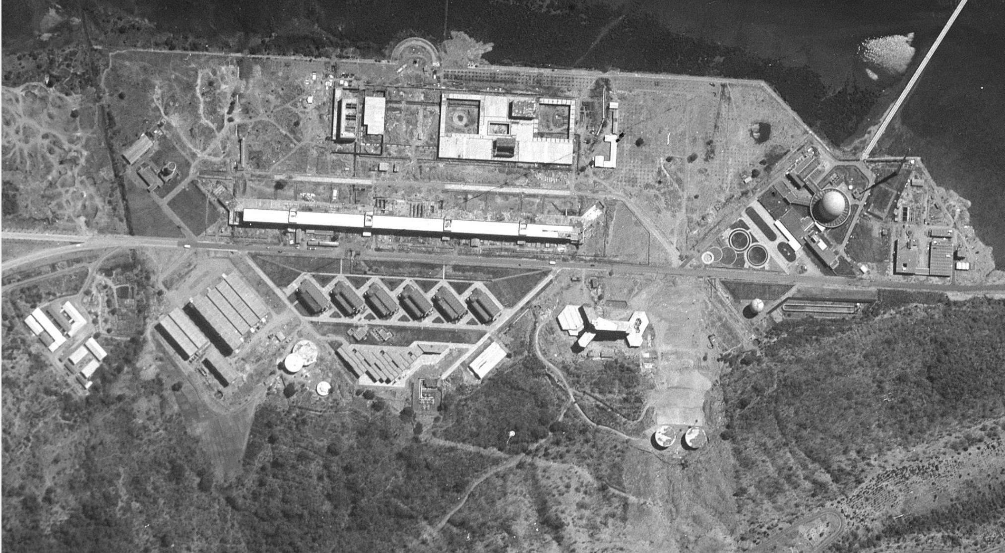
India's first reactor and a plutonium reprocessing facility, Mumbai , as photographed by a US satellite on 19 February 1966 30
