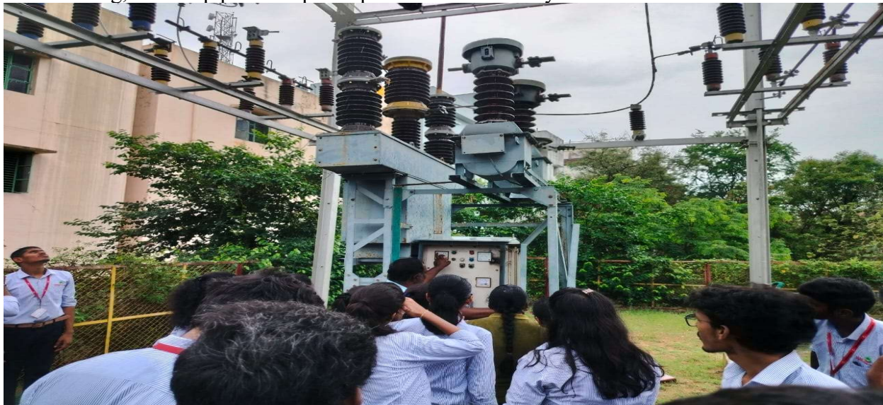
Figure 2 Demonstrating of 33kV input Circuit breaker functions with relays
