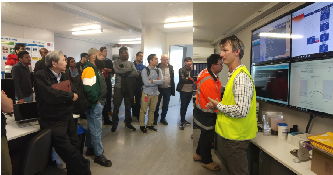
Photograph: Mr Leo Pearce (Asset) and Mr Simon Zhao (Site Manager) are describing the monitoring and control centre of the Gullen Range Wind & Solar Farm.
