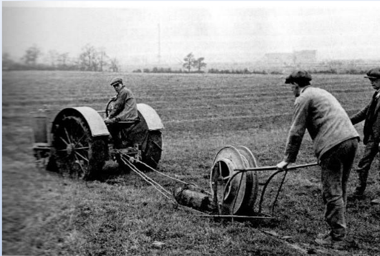
Burying Earth Wires - November 1924
