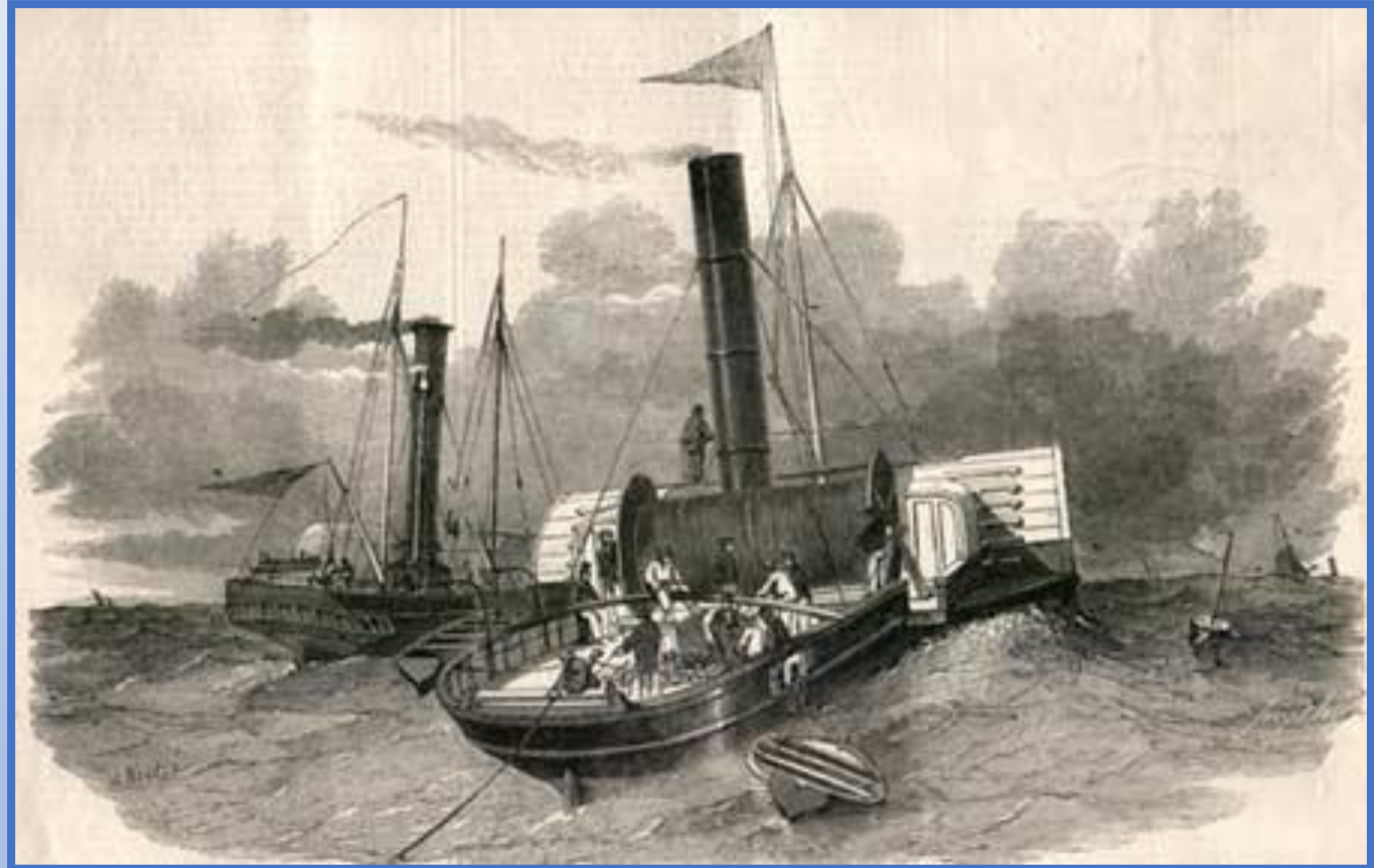
Goliath Laying Channel Cable - 1850
